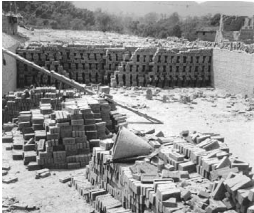
Plate 2.12 - Loading bricks into a Hoffman kiln
