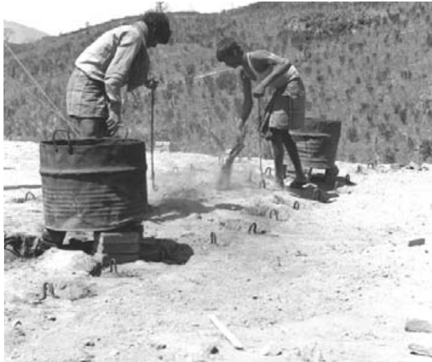
Plate 2.11 - Loading coal into a Hoffman kiln
