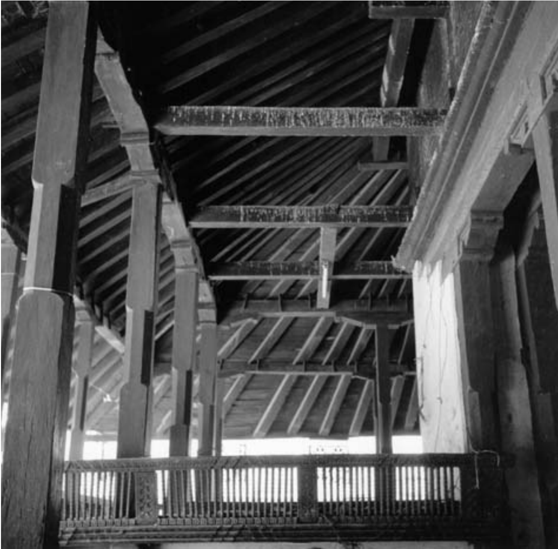
Plate 3.2 - Wood structure of the Kasthamandapa first roof
