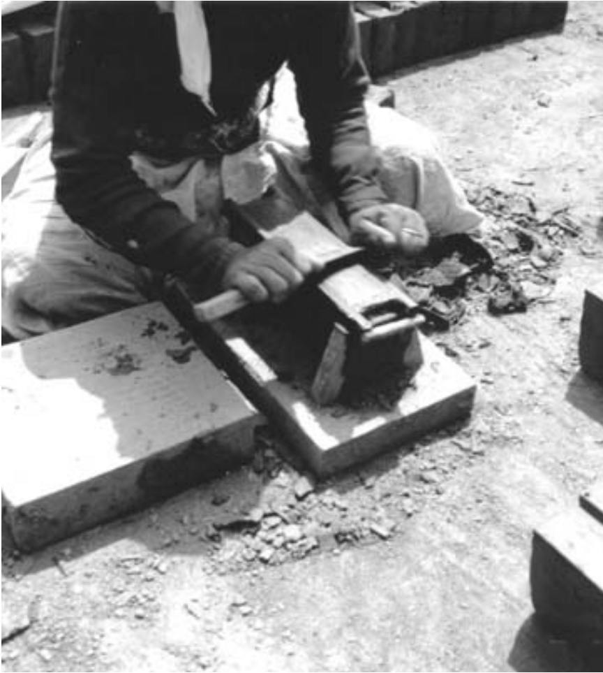
Plate 2.4 - Fair face of brick is smoothed with a knife
