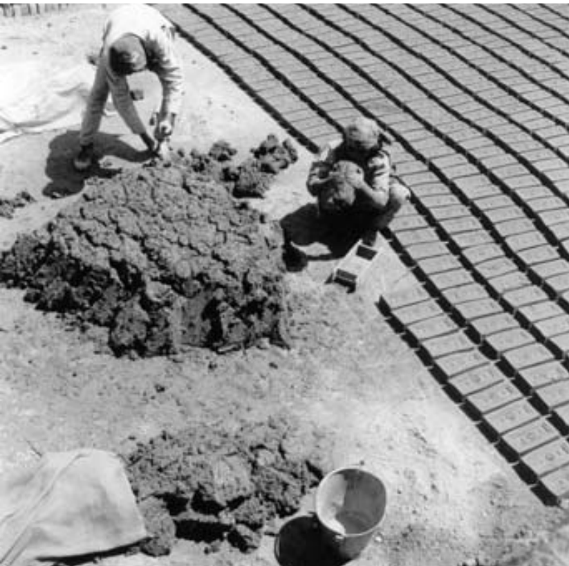
Plate 2.2 - Preparation of the clay and its insertion into the mould
